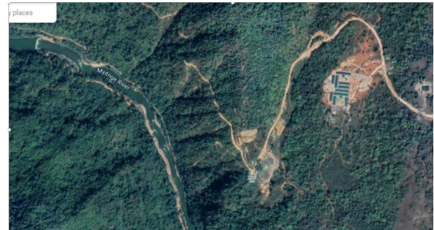
March 2020 Google image showing unauthorized construction
