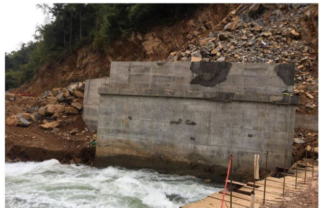
Cement reinforcement along the river's edge
