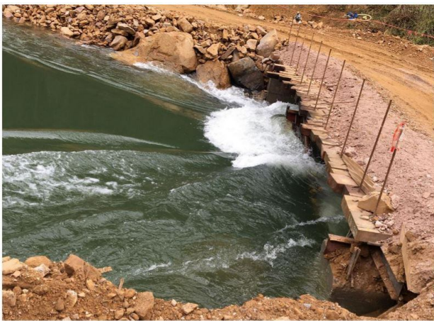
Temporary bridge built across the river
