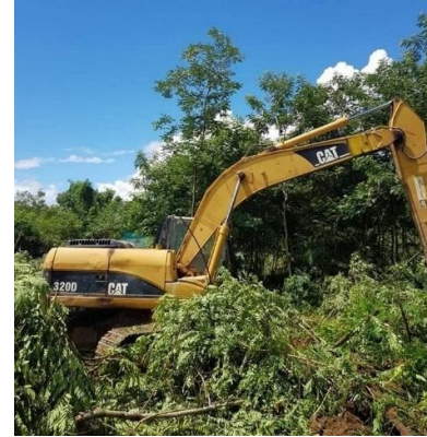
Company backhoe clearing trees
